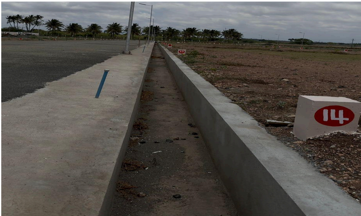
Panchayat Water Connection and Drainage System
